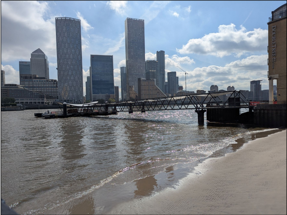
Figure 3-3: The new Rotherhithe Pier upon completion.
