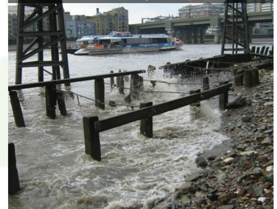
Wash and Damaged Campshed
