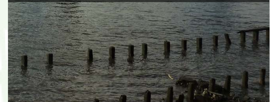
Pile stump obstructions
