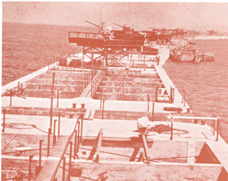
Construction of concrete caisson nearing completion in the London docks.
