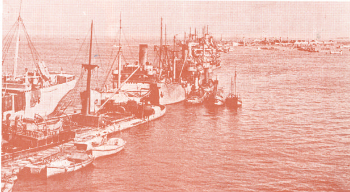
Blockships were scuttled to form part of the northern and seaward breakwaters.
