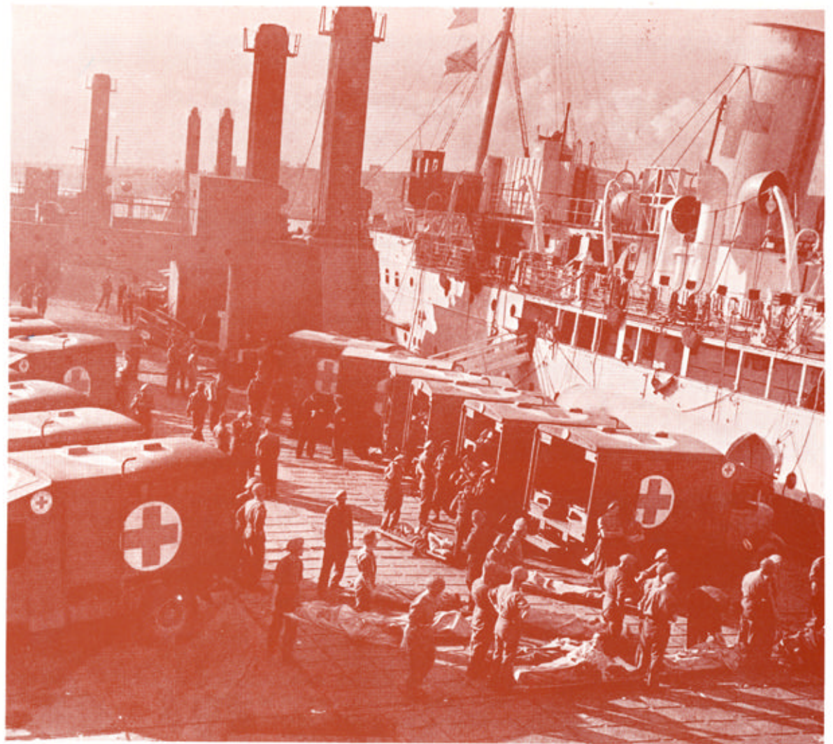
A hospital ship berthed at an LST pierhead.
