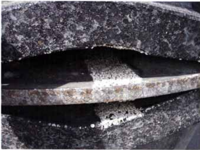
Figure 6: The barnacle growth extends the full length of the flutes
