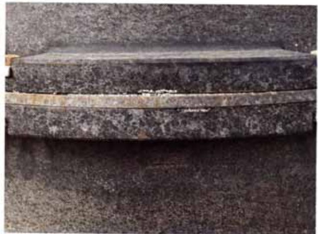
Figure 5: Barnacles filling fender vent flutes
