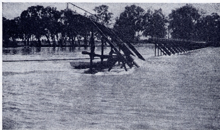
FIGURE 7. Mildura weir trestle unit moving into position in the river.
