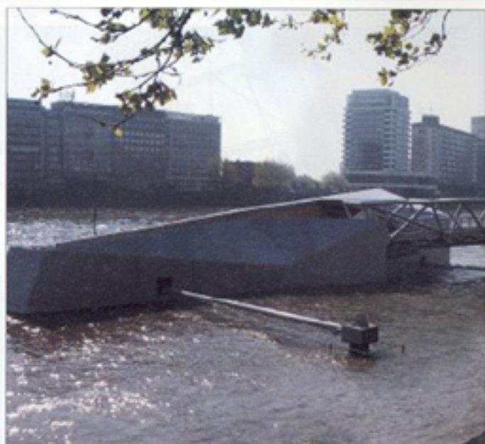
The Millbank Pier in position. Photo courtesy of Beckett Rankine.
