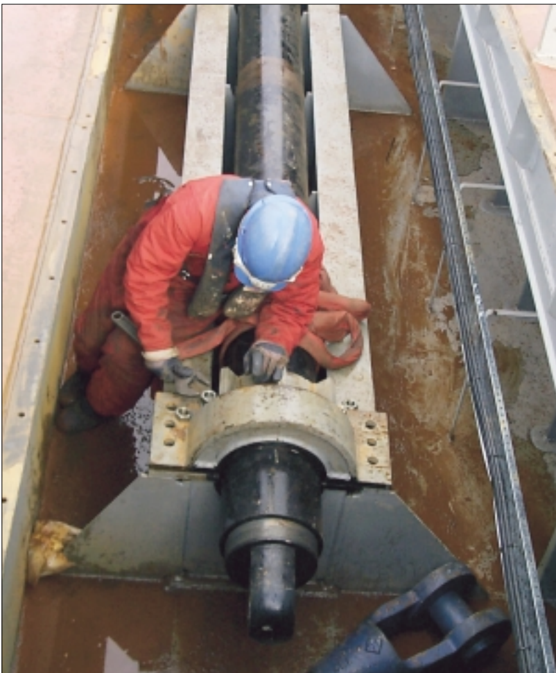
Fig 4. The main Jarret energy absorber unit mounted in the pontoon
