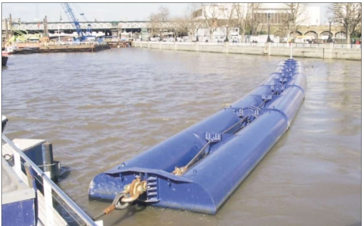
Fig 2. Floating boom carrying the arrestor cable
